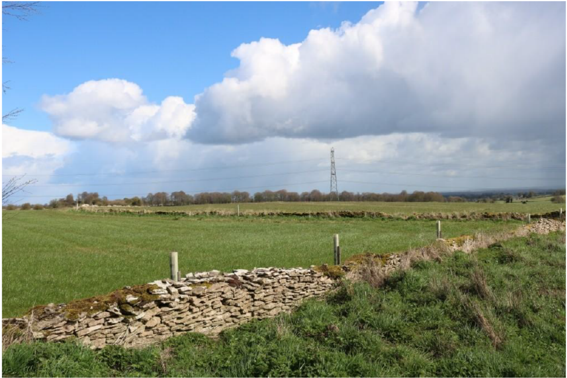
View looking north east from B4040
